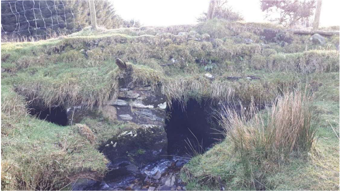
Figure 3-14: Existing Stone Bridge Crossing (WF-HF8)
