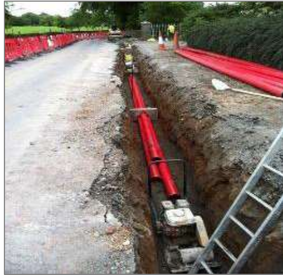
Figure 2 – Example of 110kV Underground Duct Installation
