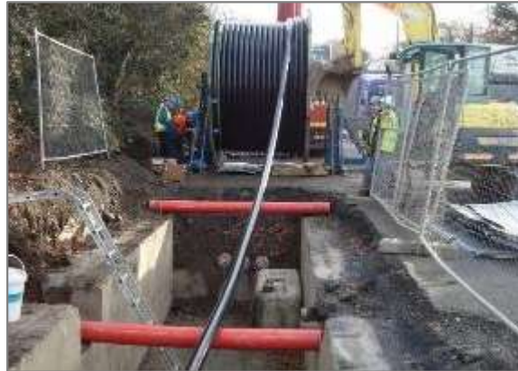
Figure 8 - HV cable pulling procedure (Drum set-up example)
