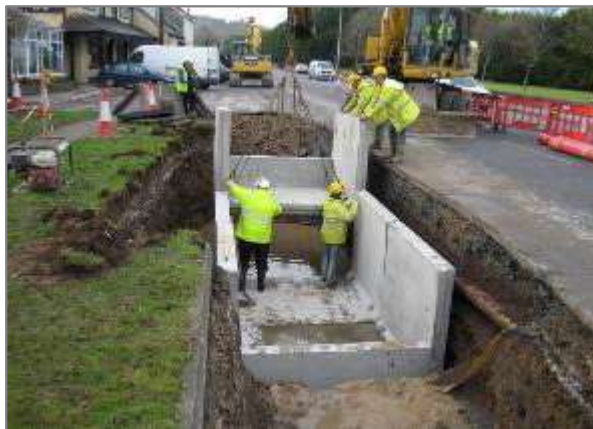
Figure 7 – Example of Joint bay under construction (pre-cast)
